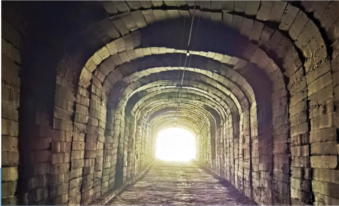
Musonoi Main Decline Ramp Musonoi主斜坡道
